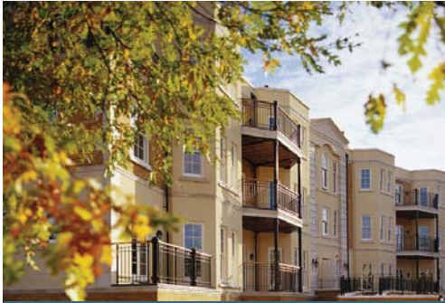
Above: Holwood, Keston, Bromley Below: Steiner Ranch, Austin, Texas
